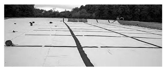
Figure 6 - Grid layout of the basin surface by strips of 1m every 10 linear meters minimum
