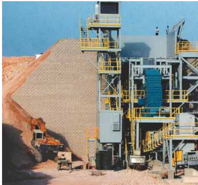
Head walls are easily assembled but provide robustness and durability in a tough working environment.
