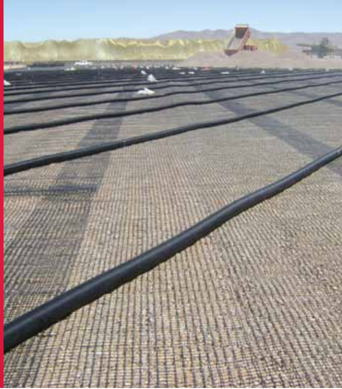
Leach pad construction with Tensar® geogrids.
