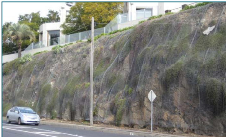
Typical Rockfall Netting Application
