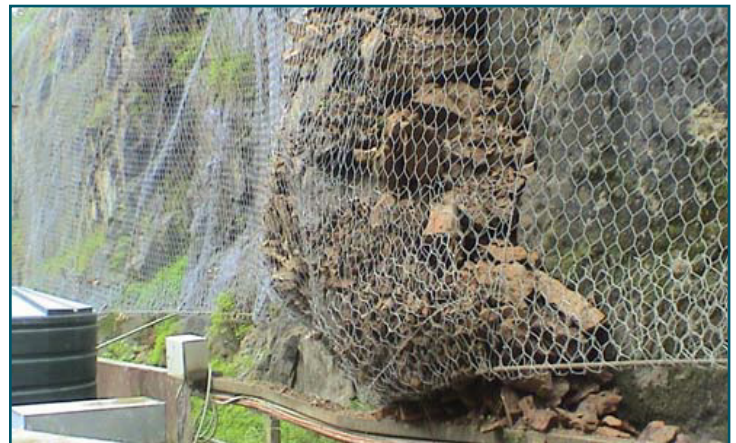
Typical Rockfall Netting Application
