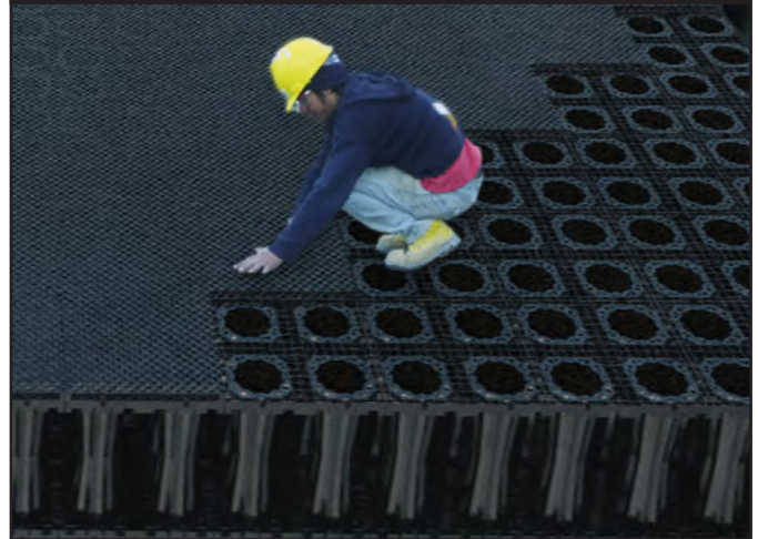
INSTALLING FLO-CELL® CAPPING LAYING OVER TANK MODULES
