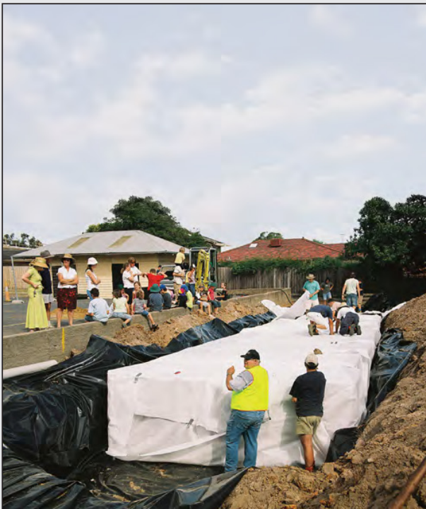
Constructed tank is wrapped in geotextile.
