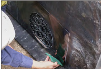
4. Prepare the area of the boot flange with a polypropylene glue
