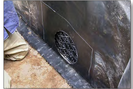
3. Cut the opening for the pipe
