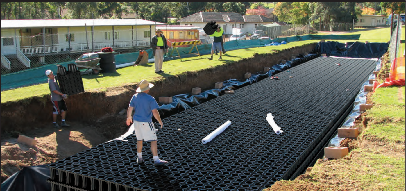
INSTALLING TANK MODULES
