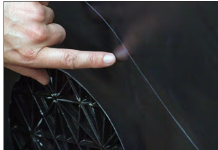
5. The area is ready when the surface is dry to the touch
