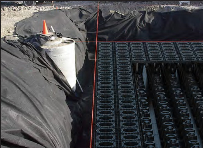
STRING LINES FACILITATE INSTALLATION OF BASE LAYER
