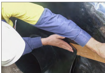
7. Mount the boot liner starting from the corner.
