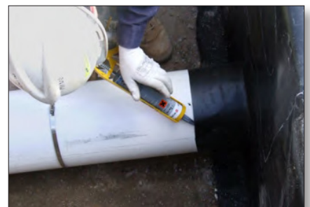
9. Apply the sealant between the liner and the PVC pipe.
