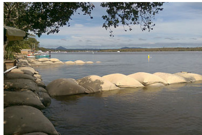
Beach view after project completion
