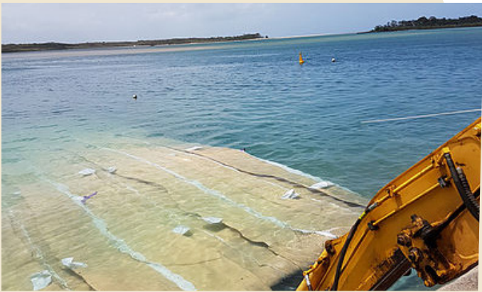
The mattresses were maneuvered into position then filled
