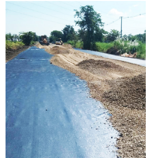
Pavement rehabilitation over expansive clay subgrade
