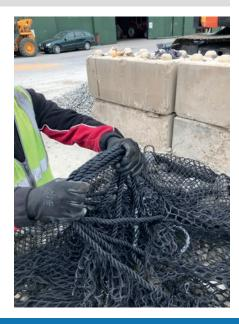
3. Pull the 8 loops up and hook them onto the centre of the telehandler. Then lift the AquaRockBag® enough to create tension on the 8 loops.
