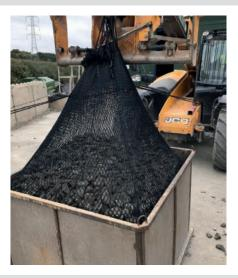
4. Two workers are needed for this and the following work step. Pull the tying rope around the AquaRockBag® in opposing directions as shown below.
