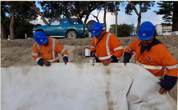
A prayer seam stitch was used to reduce the overlay, using a Class 2200 Union special sewing machine.
