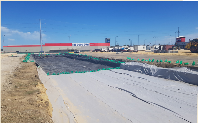
The HDPE liner and bidim® A44 as a cushion layer.
