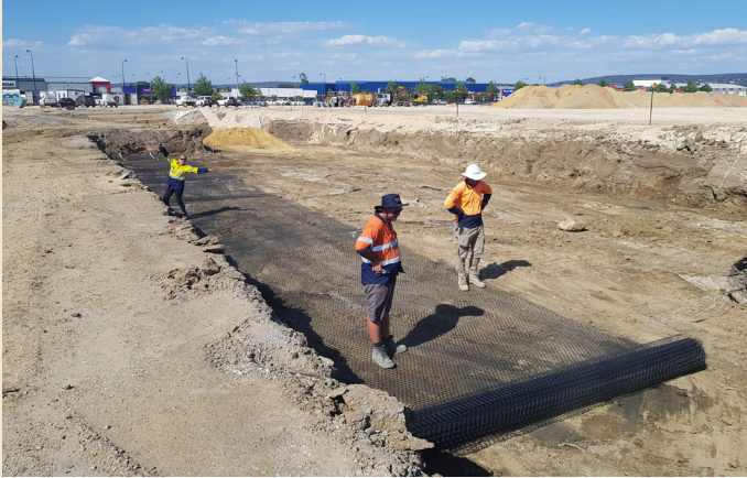
Tensar TriAx® Geogrid being installed to stabilise the subgrade.
