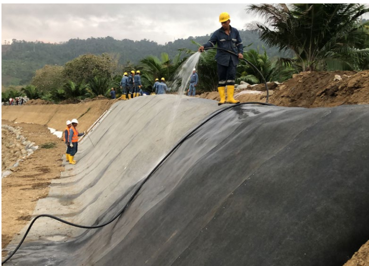
Once installation was complete, the CCX-M™ was hydrated
