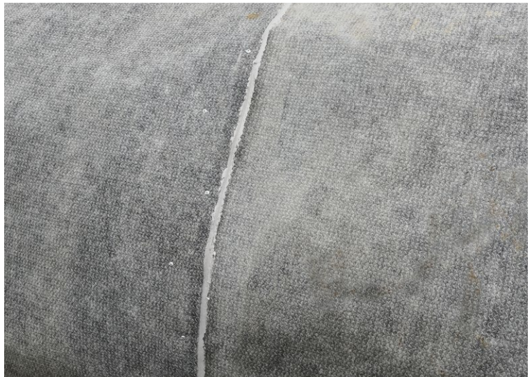
The CCX-M™ overlapped every 1.8m and secured with 30mm screws
