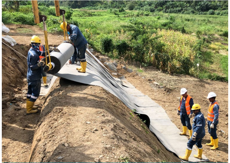
CCX-M™ installed with a boom and laid vertically
