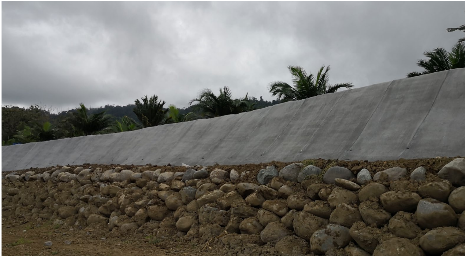
Completed erosion protection works
