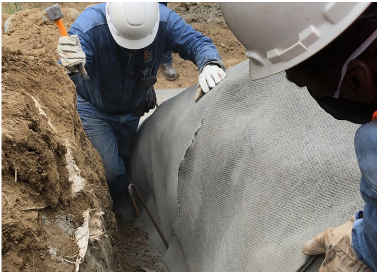
The edge of the CCX-M™ was pegged at the base of the anchor trench
