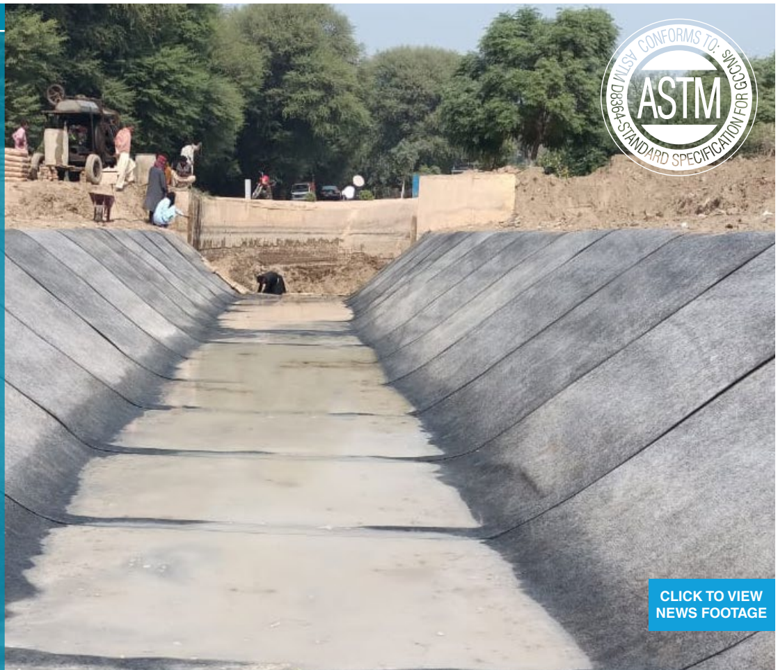
Completed canal lining works
