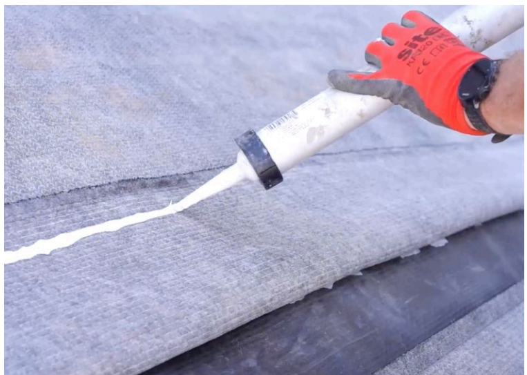
Overlapping layer of CCX-B™ sealed with adhesive
