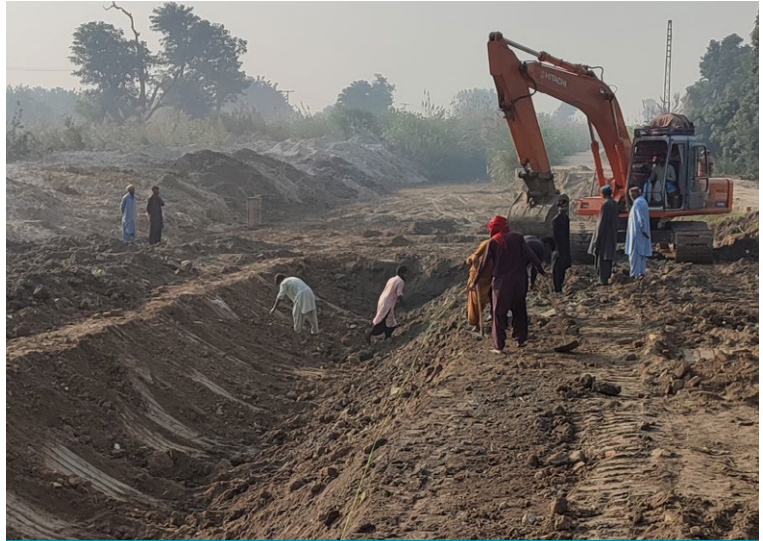
New profile excavated for CCX-B™ install
