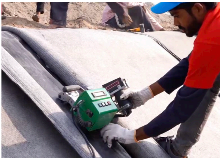
Overlapped layers of CCX-B™ thermally welded
