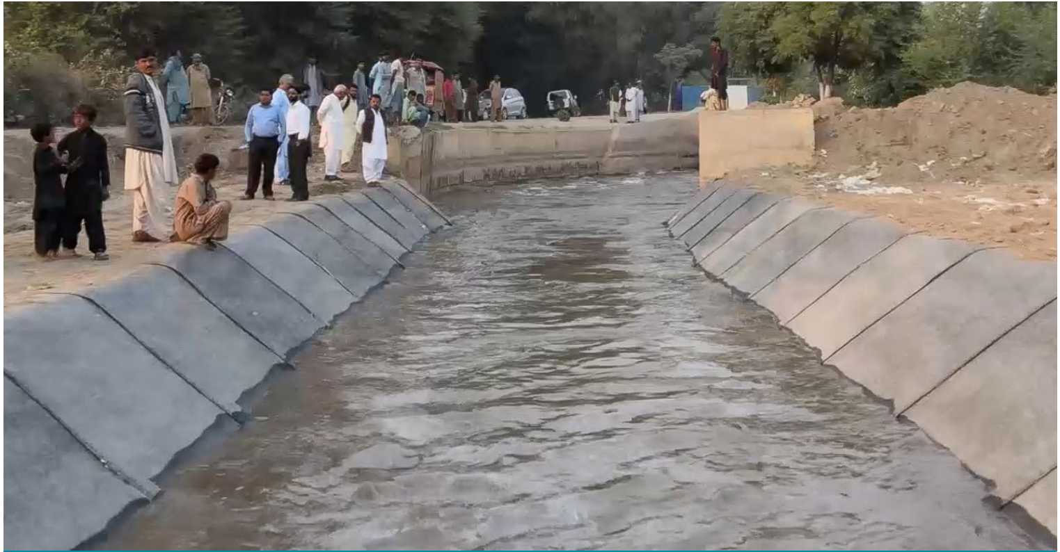
Completed canal lining works
