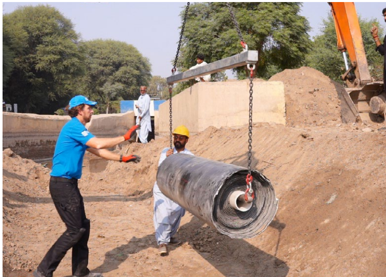
CCX-B™ Installation with aid of an excavator and spreader beam
