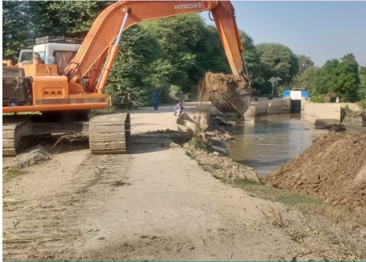
Existing canal backfilled in preparation for profiling
