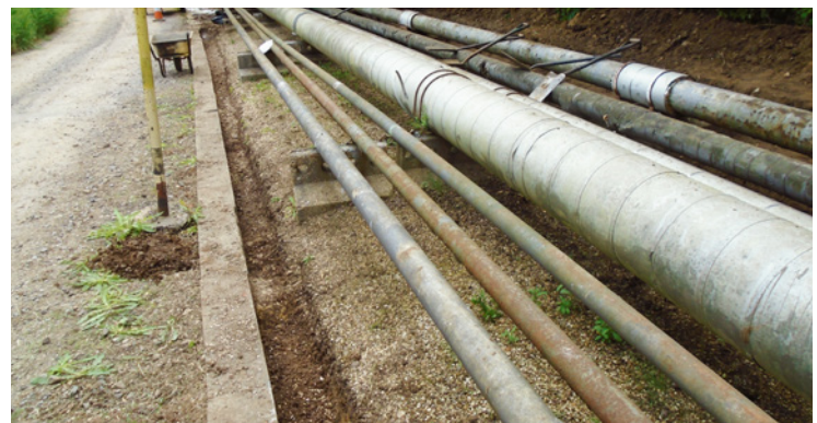
Prepare anchor trenches around perimeter edge for CC termination
