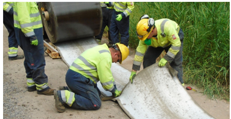
CC cut to required length
