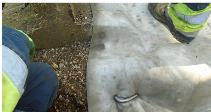
CC fixed to substrate and existing infrastructure
