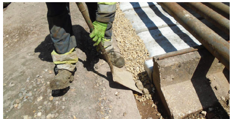
Backfill anchor trench
