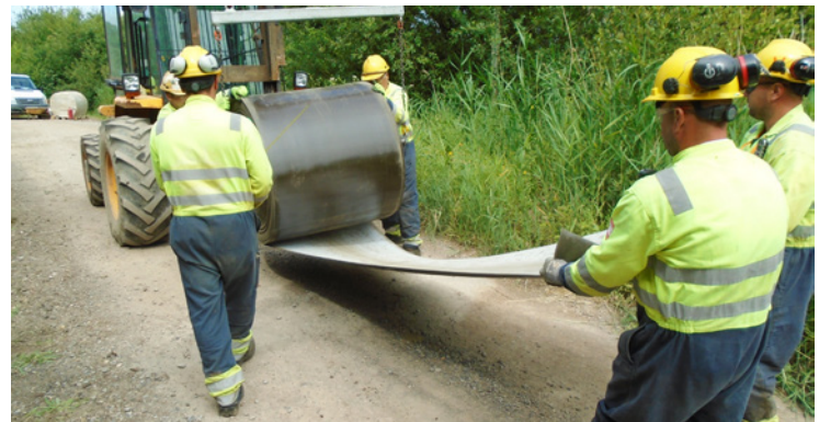
CC deployed from spreader beam
