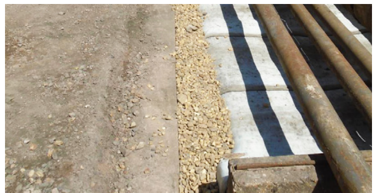
Secure all perimeter edges
