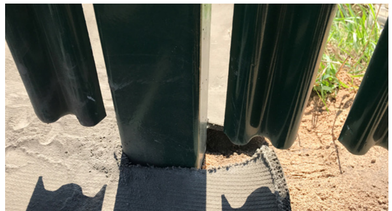
CC cut to fit around existing upstands
