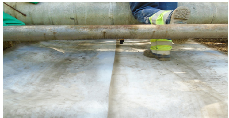
CC can be easily and safely installed around existing infrastructure
