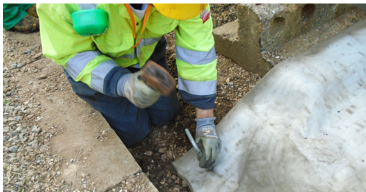
Fix CC to substrate using ground pegs and lump hammer
