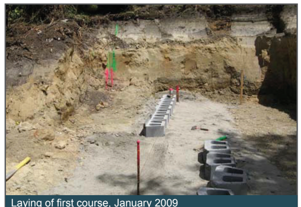
Laying of first course, January 2009
