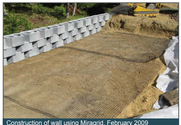
Construction of wall using Miragrid, February 2009
