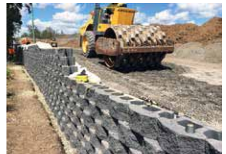
Compacting the granular reinforced fill behind the segmental block wall
