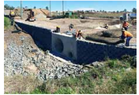
Keystone® Compac block wall at height of concrete culvert head wall
