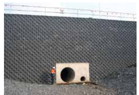
Completed reinforced segmental block wall at culvert location
