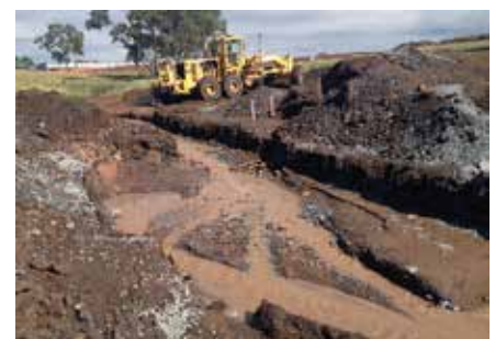
Soft soil conditions through culvert area
