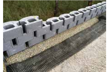
Reinforced segmental block wall showing Keystone® Compac block, Miragrid® 8XT geogrid and drainage layer components
