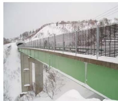
High winds can bring havoc to transport infrastructure and Parafence windbreaks are used increasingly to reduce potential danger and damage – and to provide relatively unobtrusive screening on roads, railways etc.
